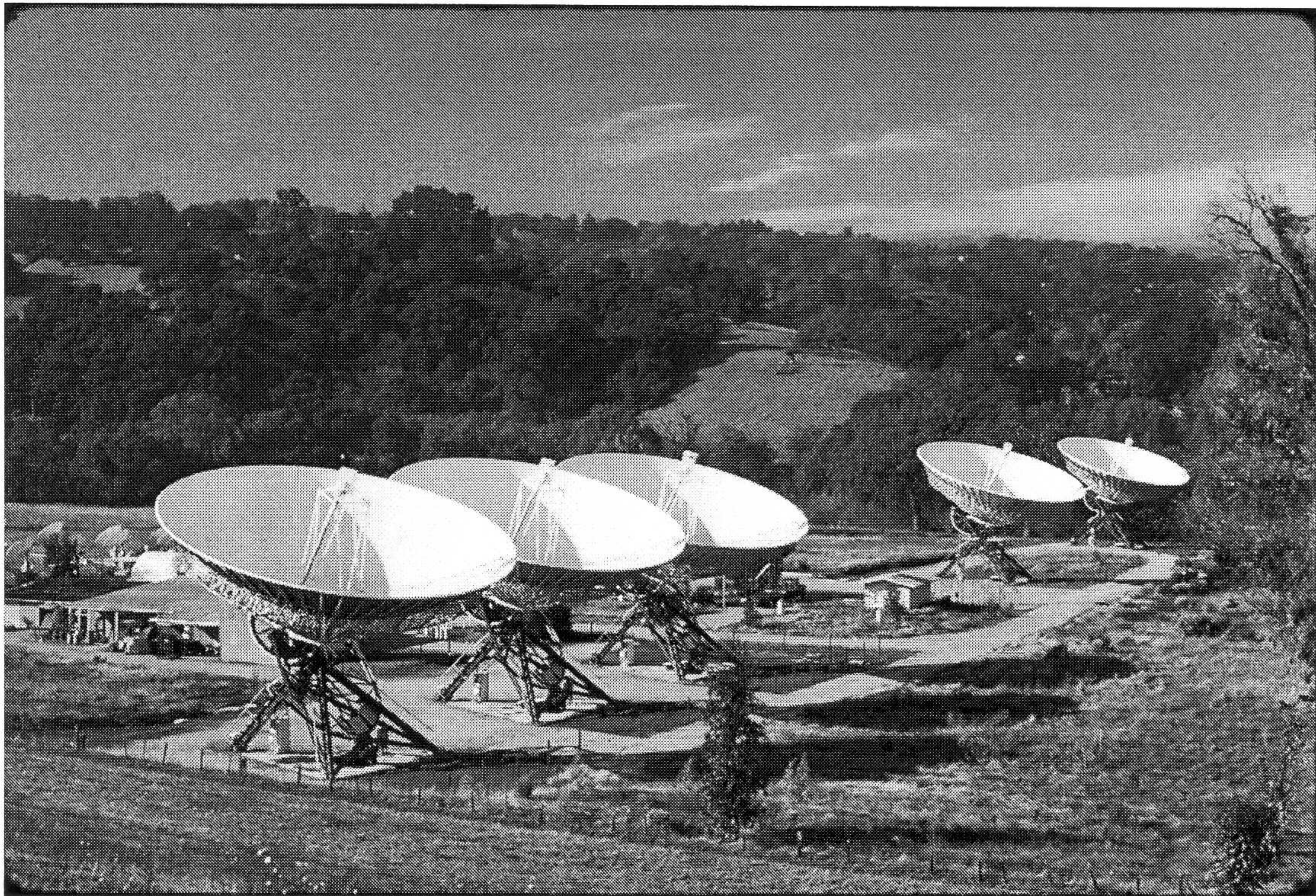
The Stanford Five Element Array, consisting of five 60-foot dishes, combiner building, and control room. Construction began in 1966.
