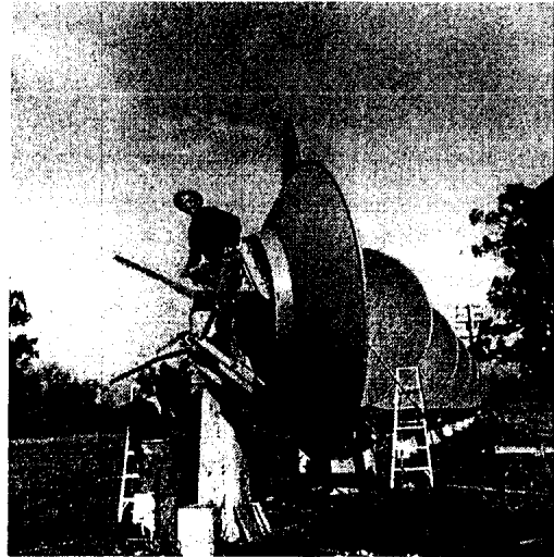
Construction of the 32-dish array, 1955-1959
