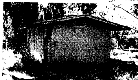
View looking west, 9/2004 Antenna Combiner Shed, 500 sq. ft. Fully intact, but roof needs repair.
